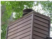
Minor Defect Acceptable Flue/Flue Cap: Metal~ Chimney crown rusted-needs primed and painted
