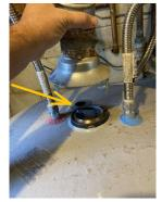
Acceptable TPRV and Drain Tube: CPVC drain line
