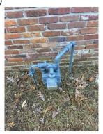
Acceptable Main Gas Valve: Located at gas meter
